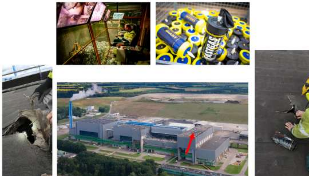
Figure 2: Cilinder flew through roof plating out of the bunker outside (Dutch EfW plant).
